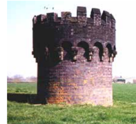
10 Air shaft turret for Sodbury rail tunnel. One of 6 in the LCA.
