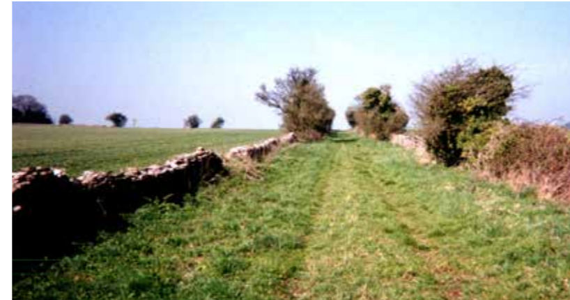
9 Green lane near Lyegrove (Tynning Lane). Dry stone walls in poor condition.
